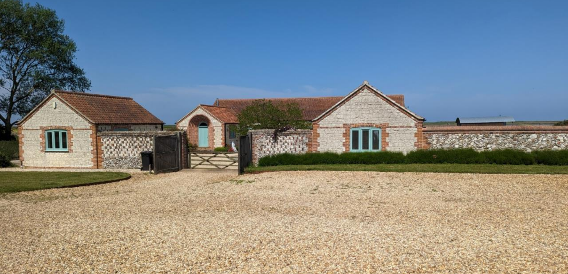
Existing dwelling and outbuildings
